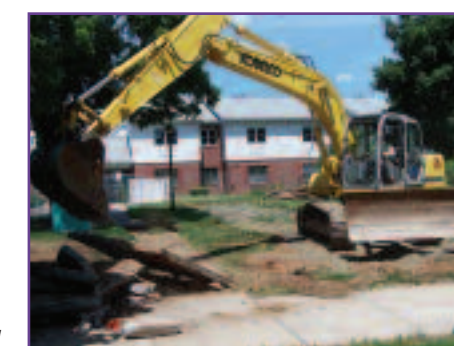
Construction is underway at Elim Park!
